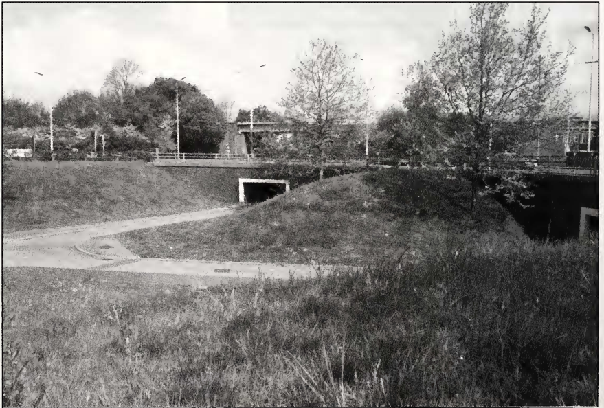
Figure 3. Twin Bridges roundabout south (site 14) was representative of several roundabouts which were sunk below the level of the road and dissected by one or more pedestrian/cycle paths accessed via subways.
